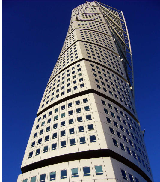
Turning Torso (Malmö, Sweden)
