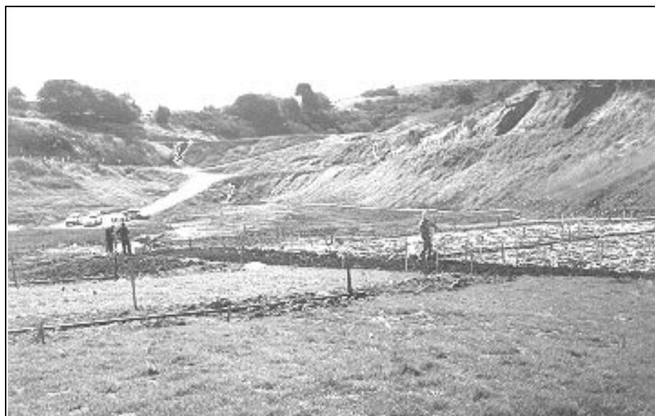
This view shows the area of work at the West Coast field site.
