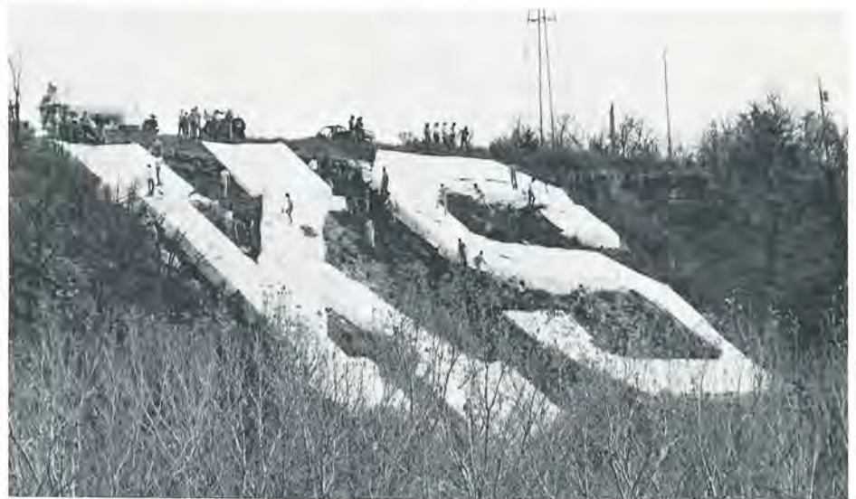
Engineering students were out again this year for their annual whitewash of K-Hill. They used 14 sacks of Portland cement, 14 sacks of lime, 750 gallons of water and an assortment of brooms, hoes, barrels and buckets for the cleanup of the 80-foot by 60-foot concrete letters.
