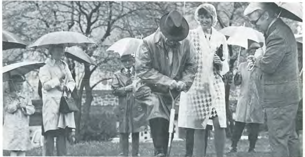
DEAN EMERITUS M. A. DURLAND who headed the college of Engineering and Architecture (1949-1961) turned the first shovel of dirt during April 29 groundbreaking ceremonies held in a heavy downpour. Ground was broken for the new $2,851,000 Durland Hall (chemical and industrial engineering). Some 150 persons — including his two daughters from California, Audrey Emmons and Mary Lee Kind — braved the rains for the ceremony. Dean Durland was honored at a luncheon following the 11 a.m. ceremonies.
