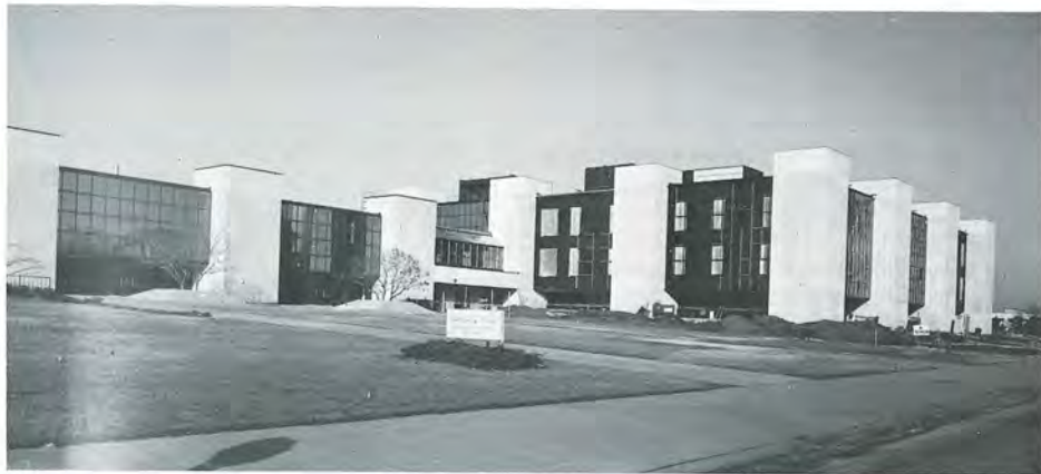
Only the finishing touches remain to be added on the facade of Durland Hall, Phase II, three-story structure at right above. The building is connected to Phase I by a lobby. The new facility is scheduled for occupancy in June, with dedication ceremonies set for early fall.
