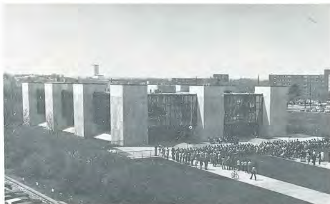
DURLAND HALL —The new home of Kansas State University's departments of chemical and industrial engineering. This $2.85 million facility, named in honor of M.A. Durland who served as K-State's dean of engineering from 1949 to 1961, was dedicated in ceremonies April 9 during the 52nd annual KSU Engineering Open House.
