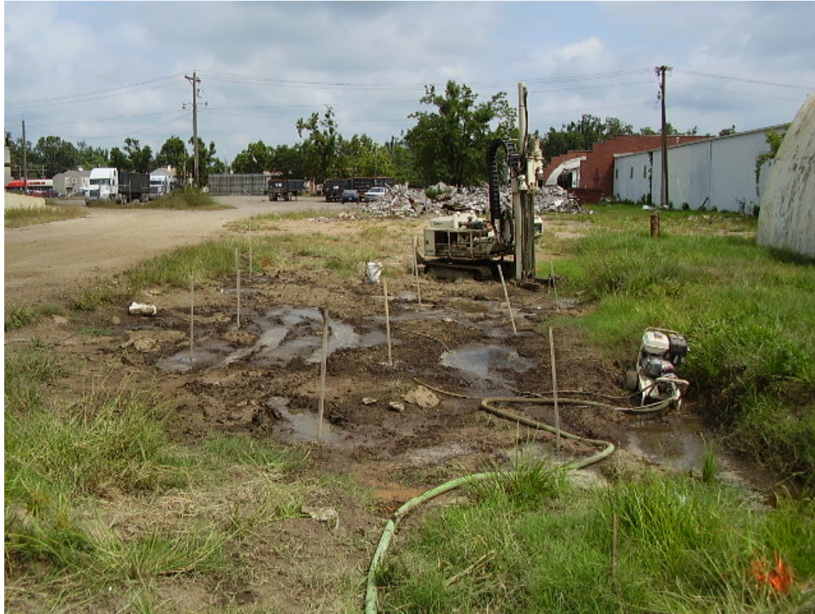
Sodium Persulfate Injection Activities
