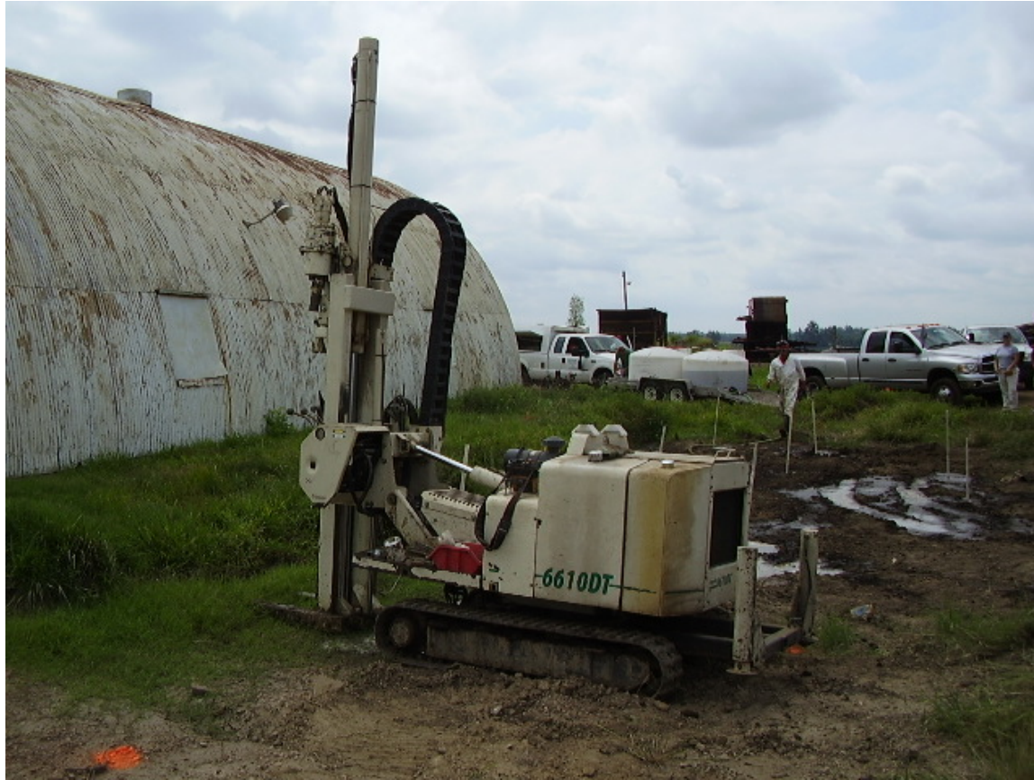
Sodium Persulfate Injection Activities
