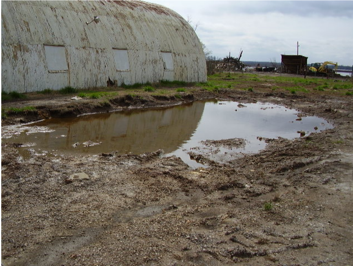
Former Chemical Blending Area
