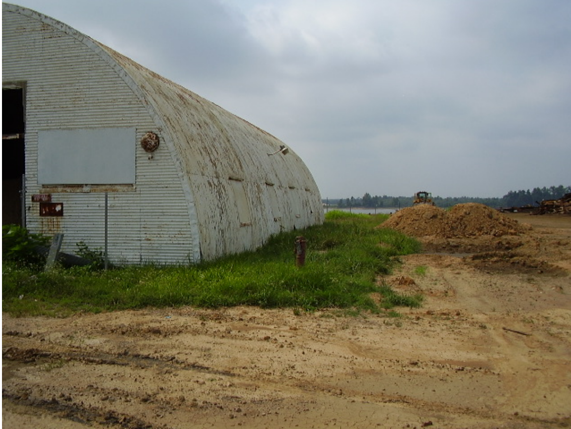
Clean Backfill in Former Chemical Blending Area
