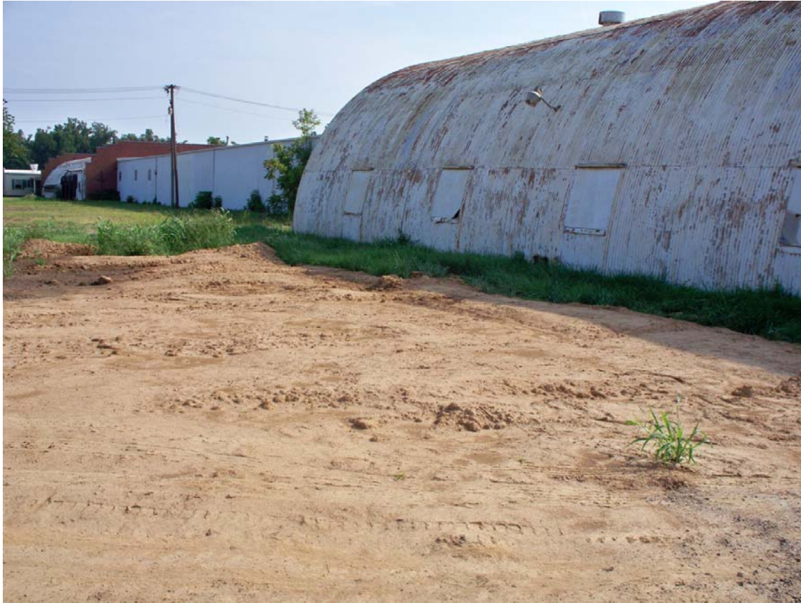
Former Chemical Blending Area
