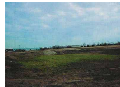
A storm water retention pond in the industrial park addition.
