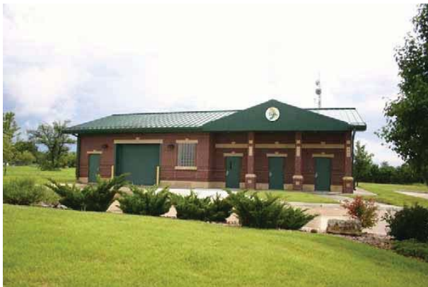
The water metering station is an attractive building in the middle of new retail development. The rest of the property is kept as greenspace. Derby
