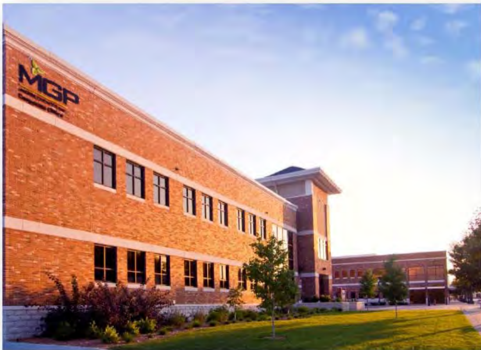
MGP Ingredients Corporate Office & Technical Innovation Center Cray Business Plaza, Atchison, Kansas
