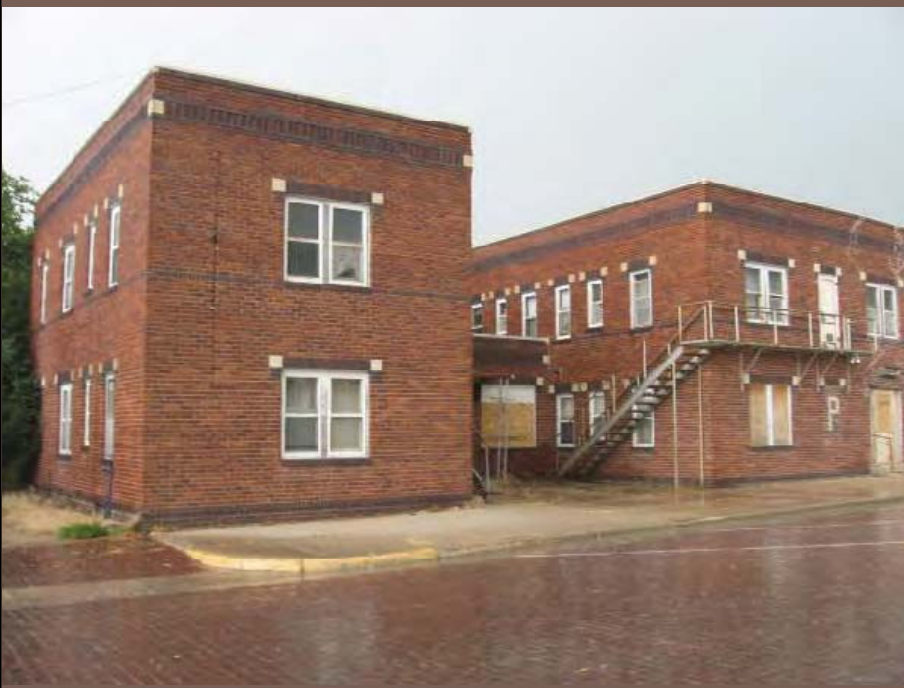
Smith Center Awarded 15K for Asbestos Abatement
