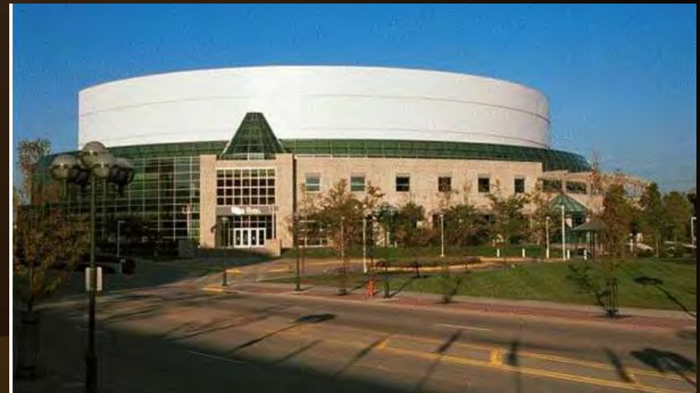
Brownfield redevelopment in Moline, IL
