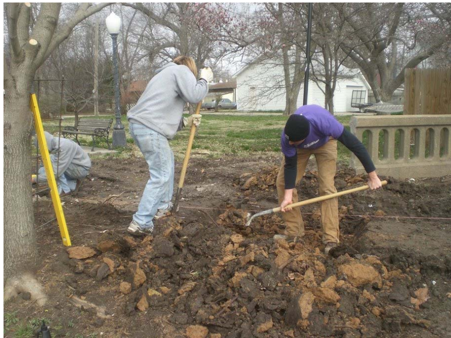
Figure 2: Students Prepare the Site by Leveling the Base Material
