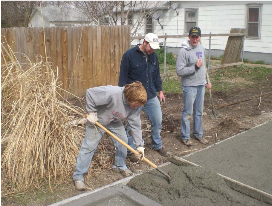
Figure 3: Students Pour and Screed Concrete to Match Existing Surface Elevation
